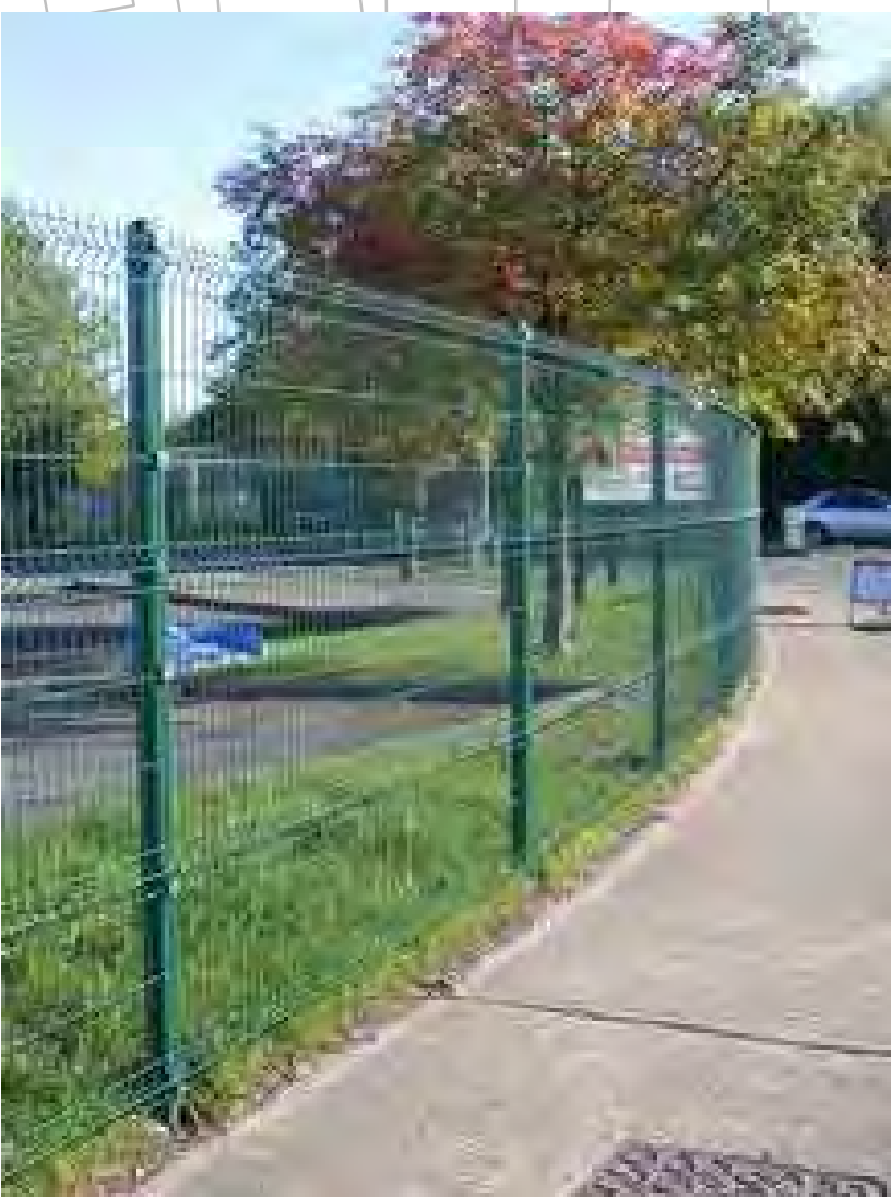
Proposed Weldmesh Fencing External, internal and ball stop fencing with gates to match. Height varies depending on location.
